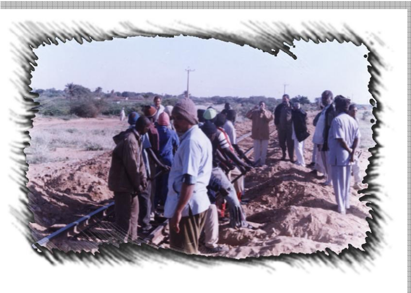
Repairing of washouts in Kosti/ER Rahad section
